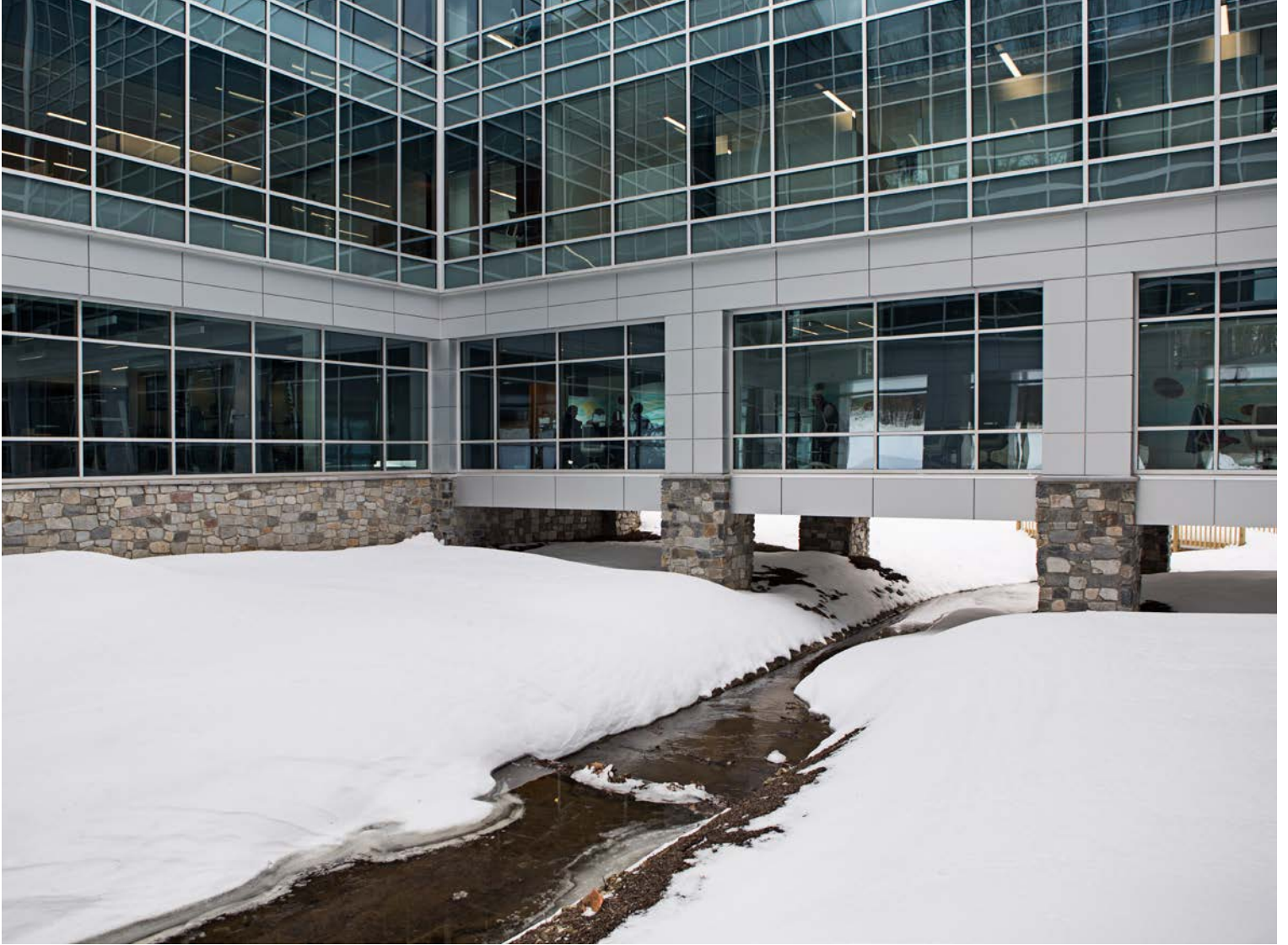
Saint-Gobain is seeking a LEED Platinum certification under the LEED 2009 Core & Shell rating.
