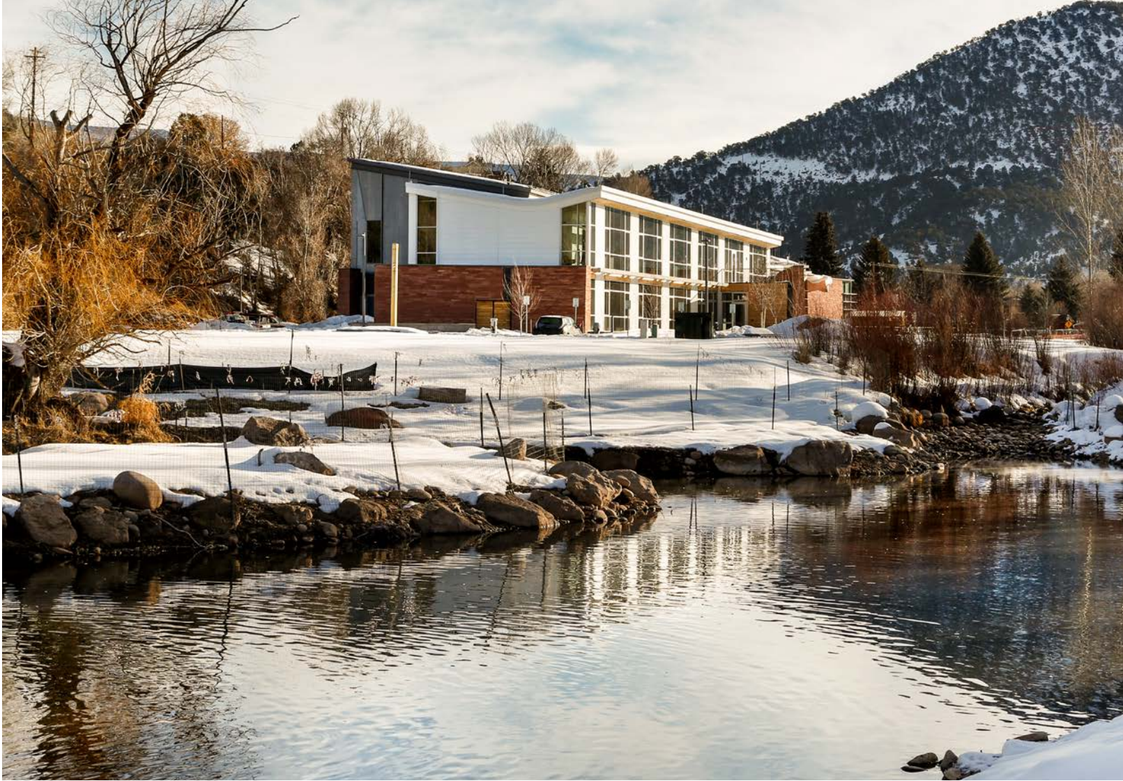
The shades on the outside of the building automatically lower when the inside temperature hits 77°F. The shades are able to completely block out the sun, but can also articulate to let in varying amounts of light.
