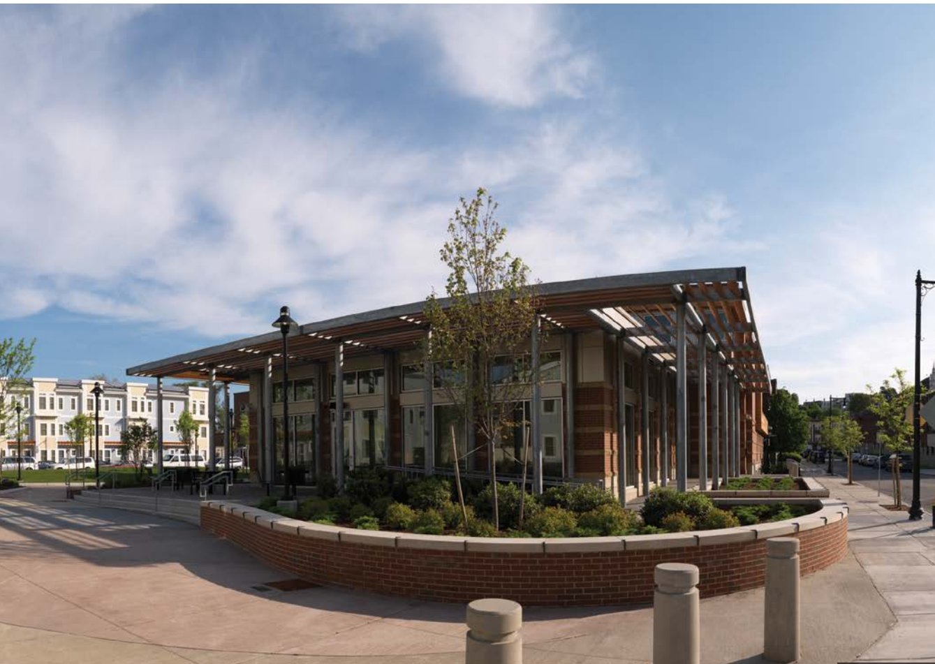
Previous spread, left page: Shiva Prakash at the Old Colony Housing project in South Boston. Right page: Beacon playground. Left: The landscaping and accompanying irrigation system around the buildings and the Joseph M. Tierney Learning Center was designed to require very little watering and maintenance.
