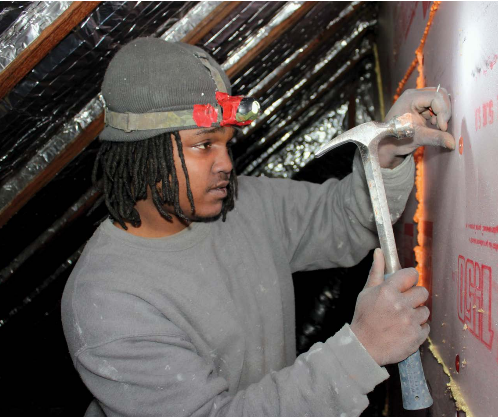
Amir Mans found a new career weatherizing houses through YouthBuild.
