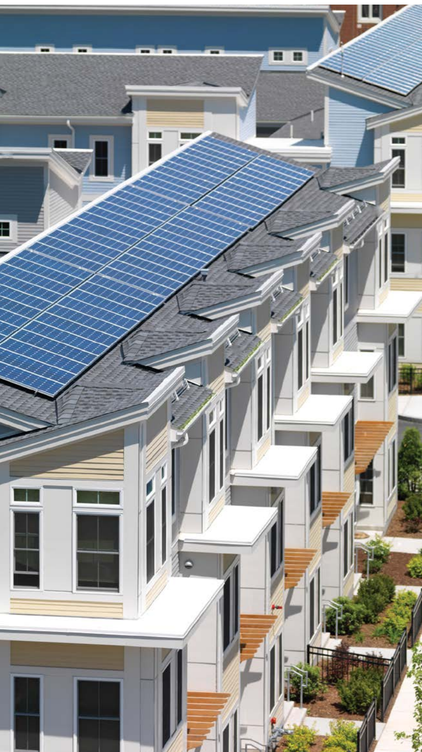
Most of the townhouses have photovoltaic panels that provide electricity to the site.
