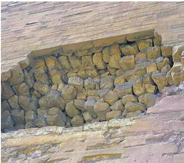
Left: A gash in the side of one of the pyramids shows a combination of irregularly cut quarried limestone blocks surrounded by tight-jointed, cast-in-place geopolymer blocks. Right: Curved, perfectly aligned joints between these backing blocks are evidence of the blocks being cast in place rather than poured.
