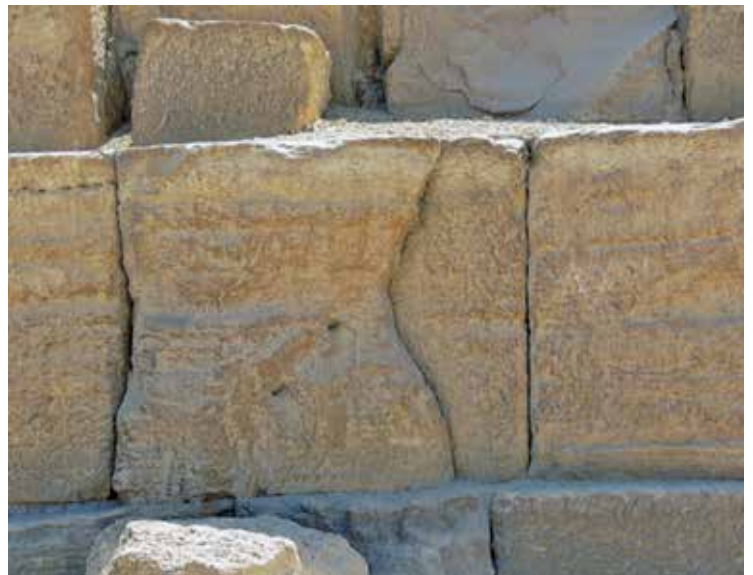
Left: A gash in the side of one of the pyramids shows a combination of irregularly cut quarried limestone blocks surrounded by tight-jointed, cast-in-place geopolymer blocks. Right: Curved, perfectly aligned joints between these backing blocks are evidence of the blocks being cast in place rather than poured.
