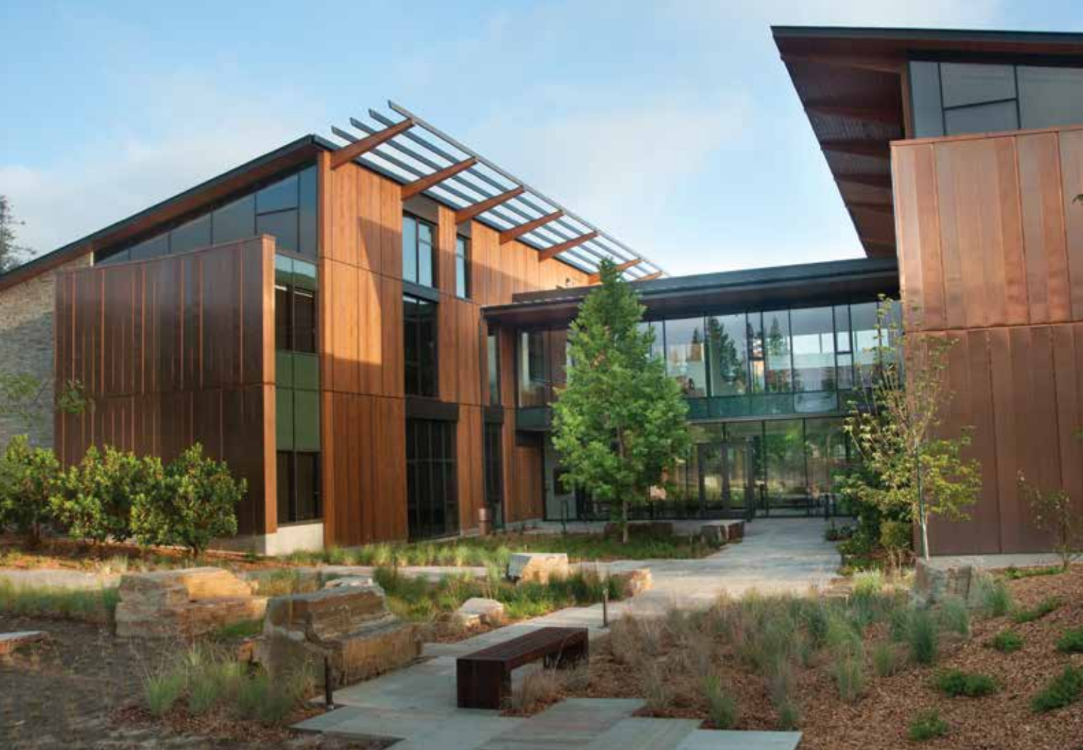
The David and Lucile Packard Foundation features 90 percent California native plants to eliminate pesticides needed by foreign plants; the landscape also uses rain gardens and permeable paving to reduce runoff and to filter pollutants.
