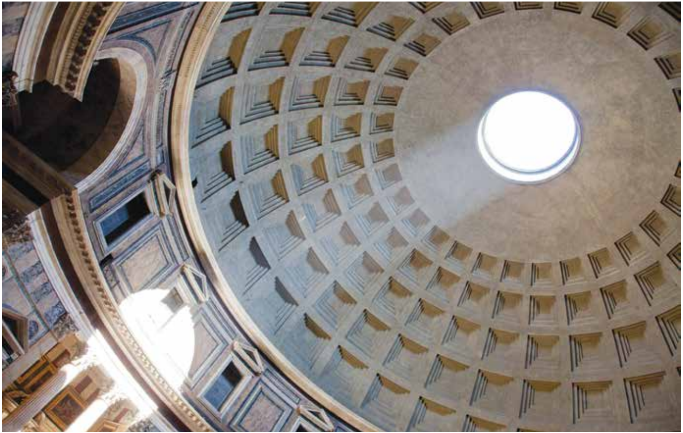
Above: The ceiling of the Pantheon in Rome—the largest unreinforced concrete dome in the world—still standing 2,000 years later. Below: Bahia Honda Bridge in the Florida Keys. The reinforced concrete deck was installed in 1938 and abandoned 34 years later.
