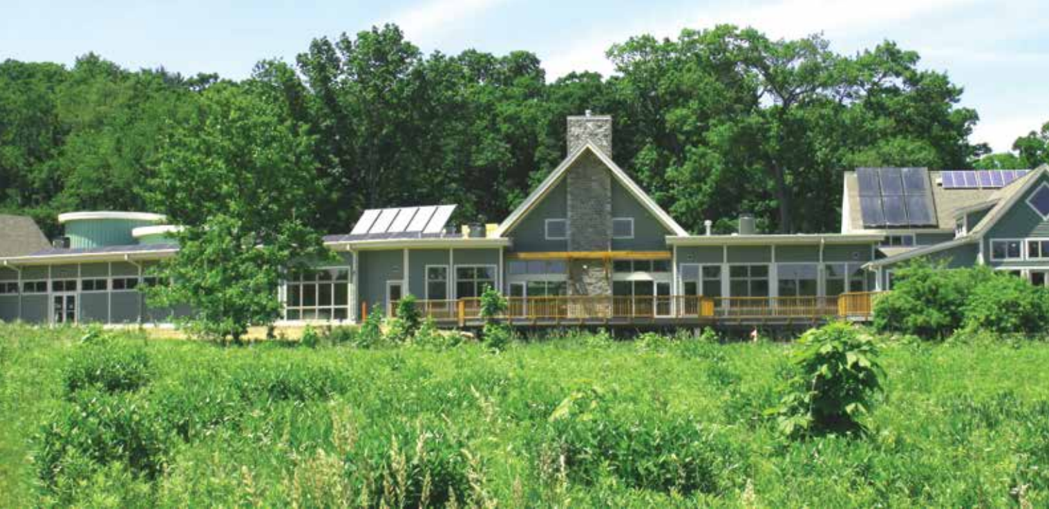
The Leopold Center's solar array meets 110 percent of its energy needs.
