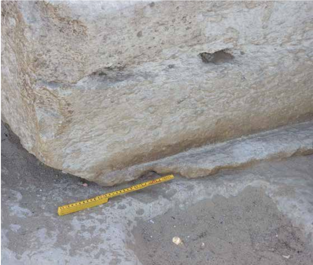
Left: A ground level block in front of the Great Pyramid of Khufu includes an irregular lip at the bottom. This lip indicates that the block was cast in place.
