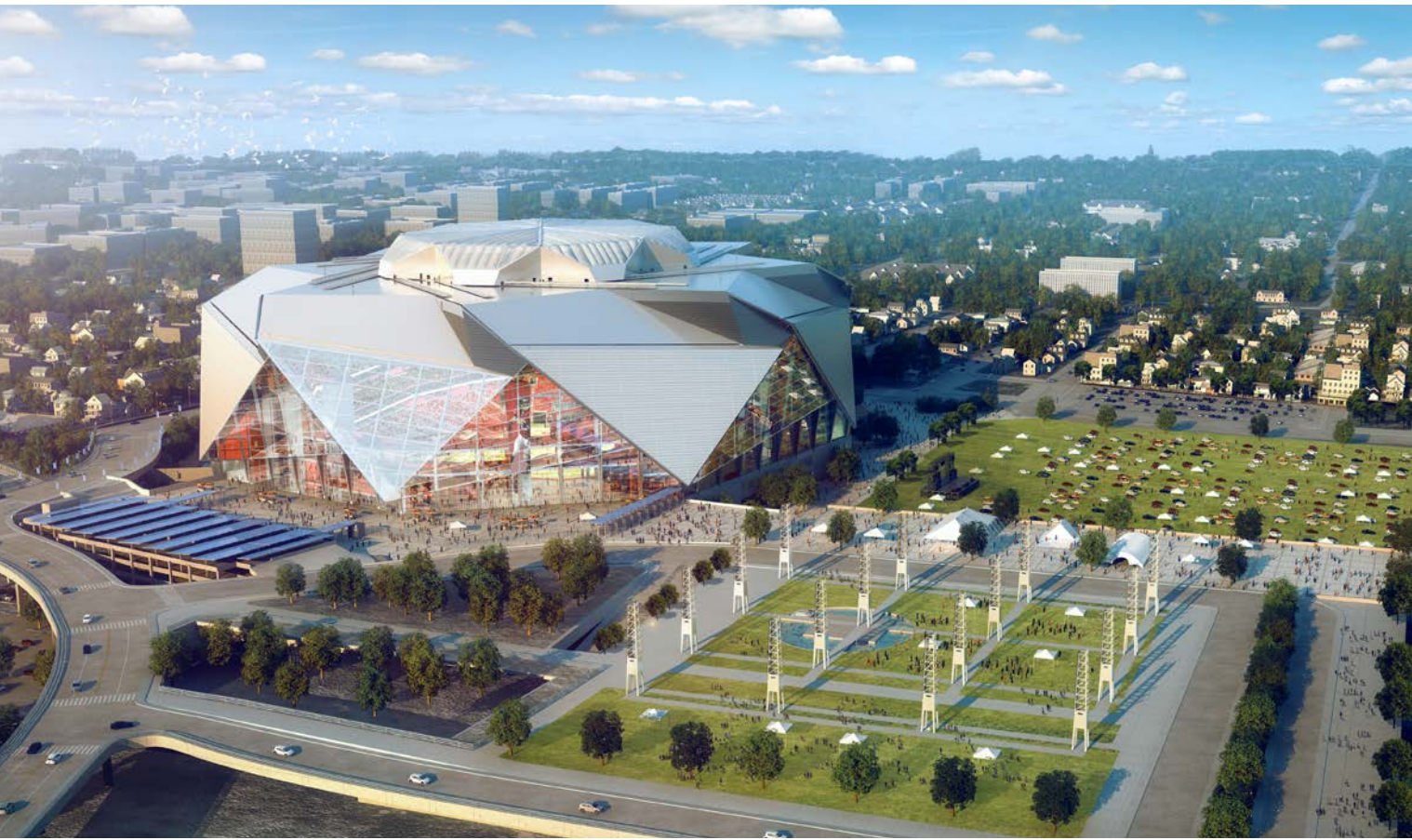
The Falcons Stadium in Atlanta will pursue LEED Platinum certification.
