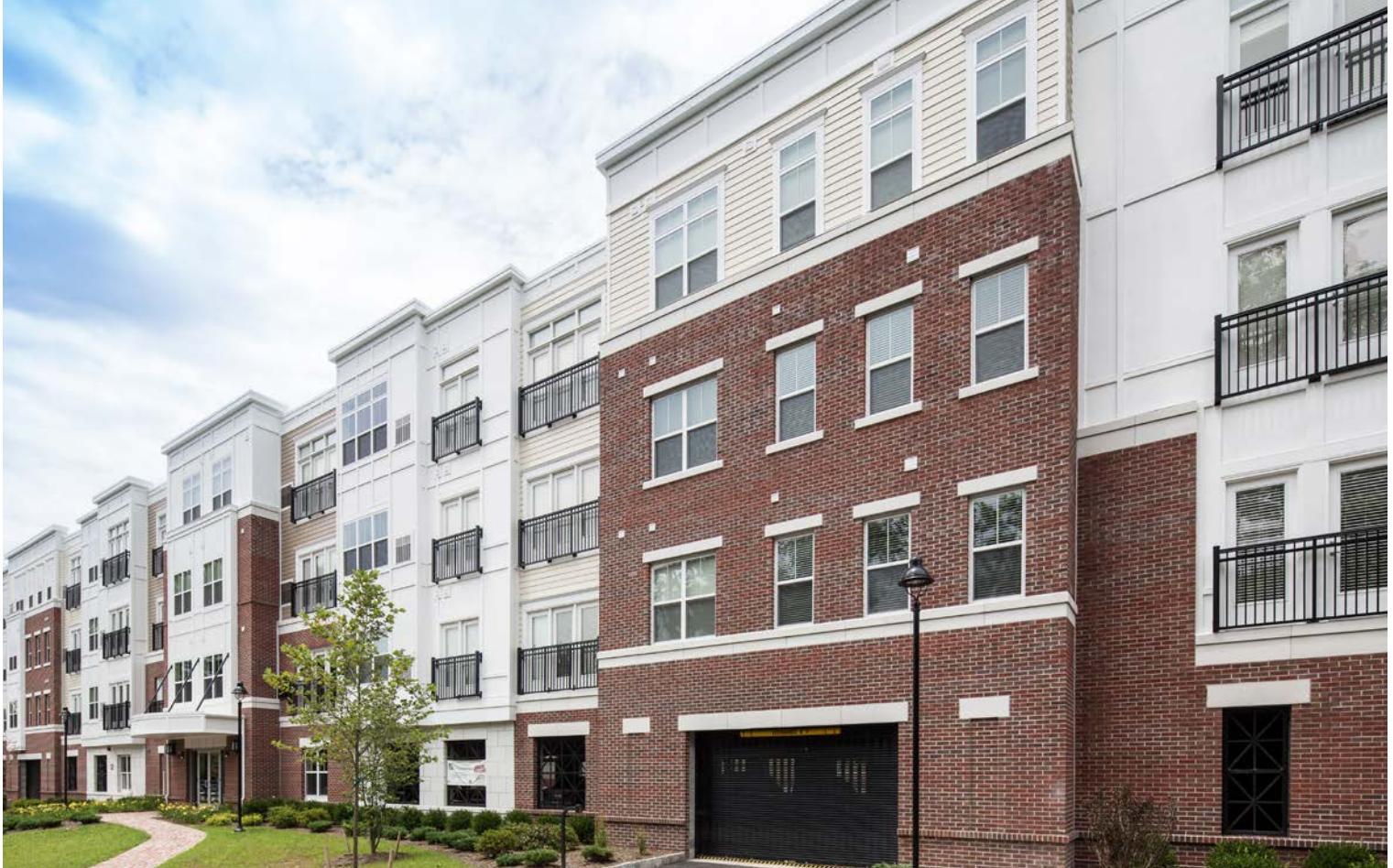
Multifamily housing such as the Station House shown here are benefitting from Fannie Mae's Green Initiative program.
