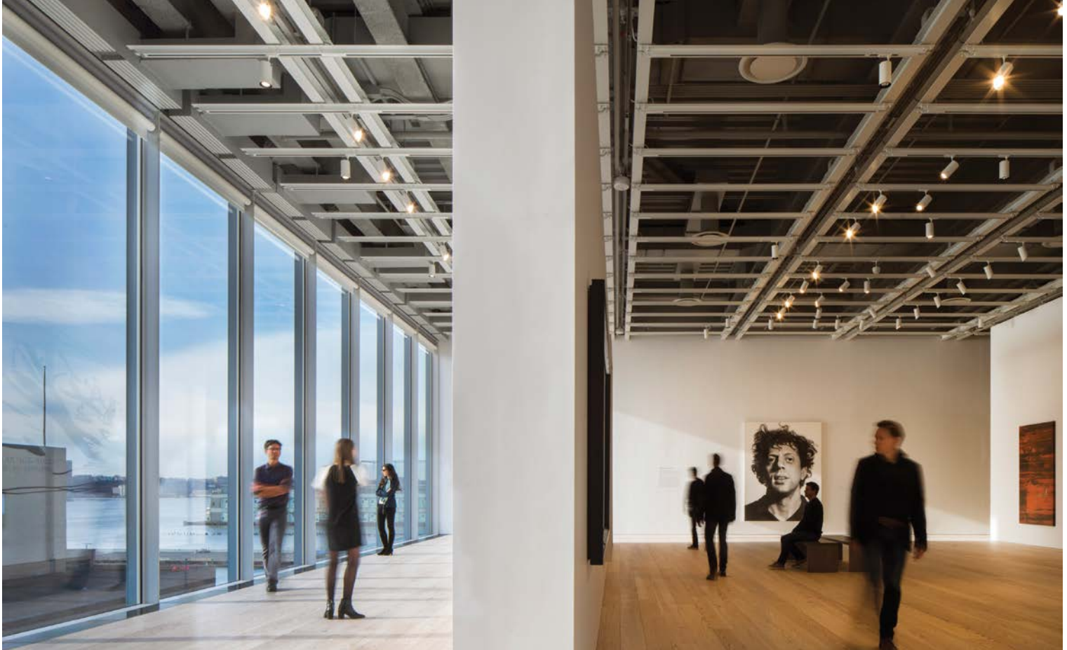
The museum's curtain wall is made with insulated glass with a three-tiered shading system.
